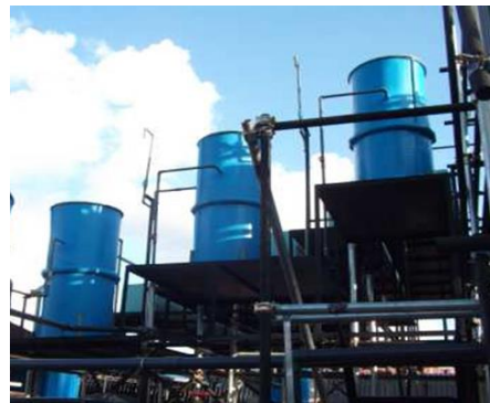
Figure 04: Up-flow Roughing Filter Unit (URFU)
