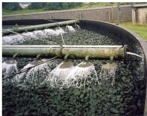
図8 礫間浄化の散水ろ床
