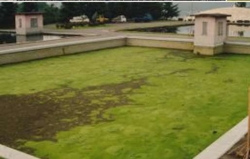
Filamentous diatom was grazed up and filamentous green algae are remarkable in warm water or in case of long filter run.
