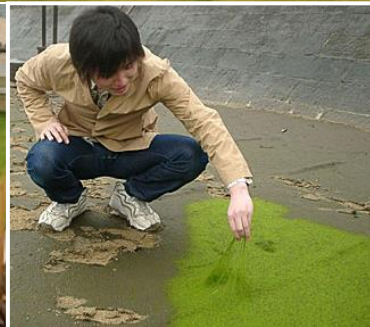
Filamentous diatom was grazed up and filamentous green algae are remarkable in warm water or in case of long filter run.
