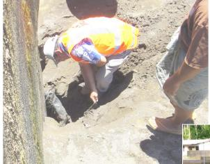
Only the sand was put on the gravel layer using a cloth to separate them.
