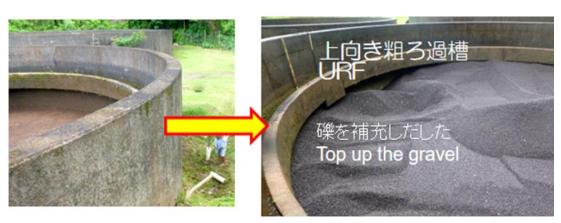
Full gravel with small crushed stones.
