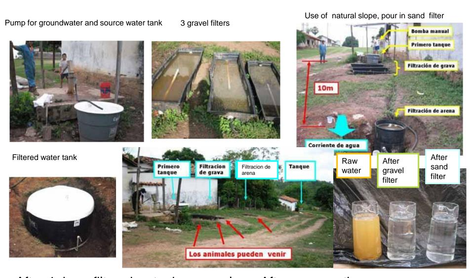
After 4 days, filtered water became clear. After one month, the water became drinkable water, in which coli-form bacteria form was not detected.
