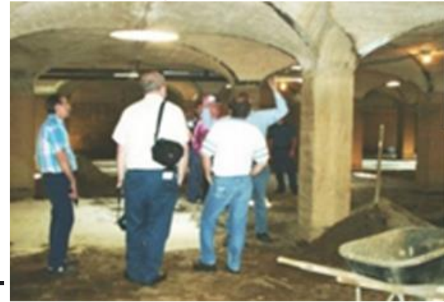
Covered filter from 1849, at Albany, NY, US Microscopic organisms play an active role in the covered filter.
