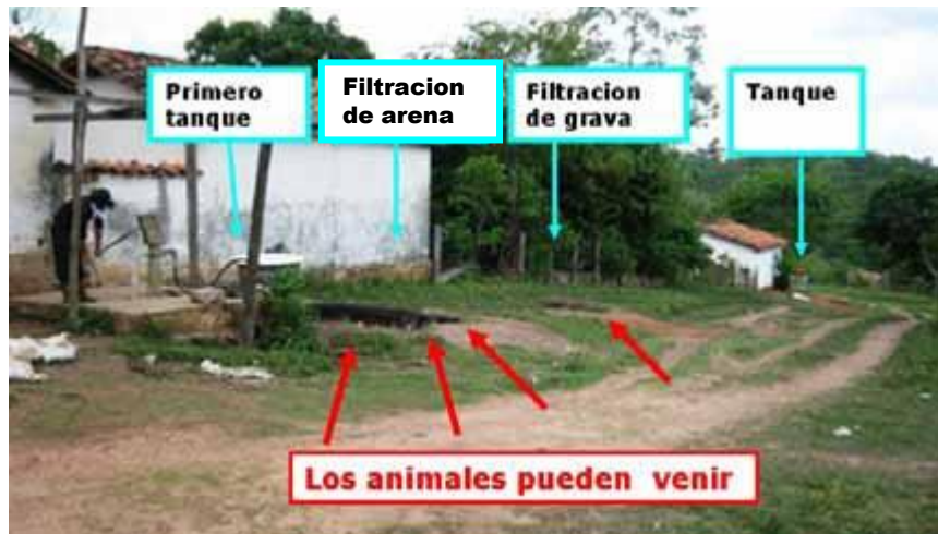
Filtered water tank
