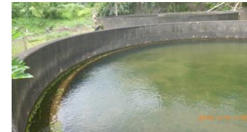
Up-flow Roughing filter:
