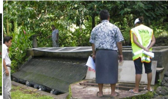
Intake Bar Screen filter
