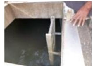
Only the sand was put on the gravel layer using a cloth to separate them.
