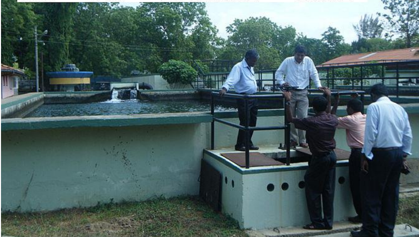
Reservoir, aerator, sedimentation (horizontal roughing filter), then slow sand filter.
