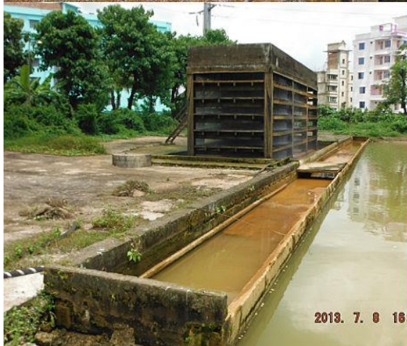
Aeration system for underground water, Chittagong, Bangladesh
