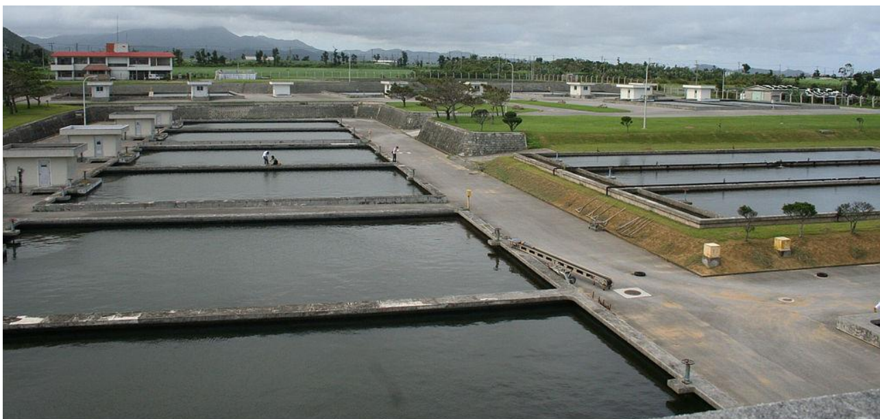
Ishigaki slow sand filter: Designed capacity: 30,160 m 3 /d
