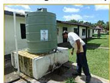
貯留槽・公共水栓 Storage tank and public tap in a village
