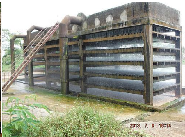
Aeration system for underground water, Chittagong, Bangladesh
