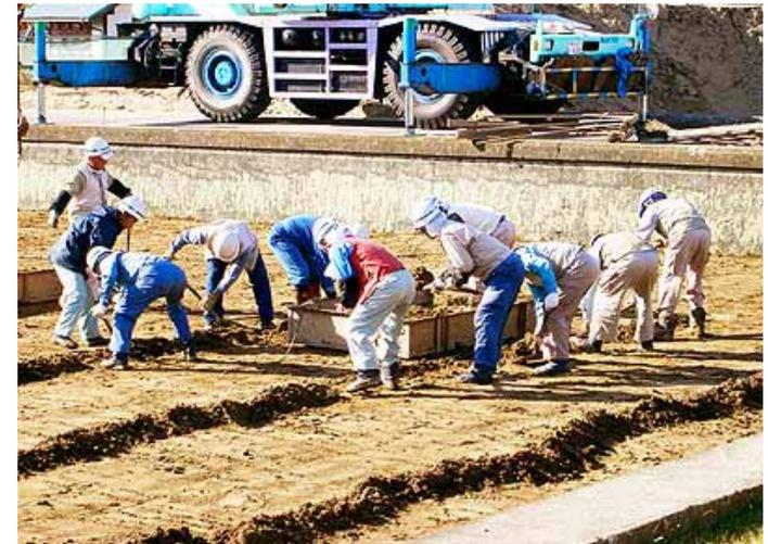
Filtrate water becomes clear water in 10 days. In summer, scrapping of surface mud is not necessary.
