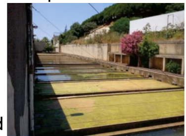
Rapid sand filter at Dbayeh: frequent back washing is needed to prevent clogging.
