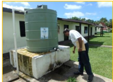
BALANCE Tank : over-flow to keep gentle flow for EPS
