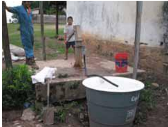
Pump for groundwater and source water tank
