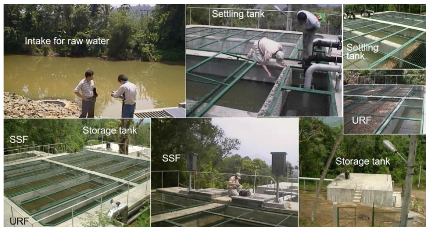
Fig. 19-1. New WTP by EPS supplied 140 m 3 per day of safe water.
