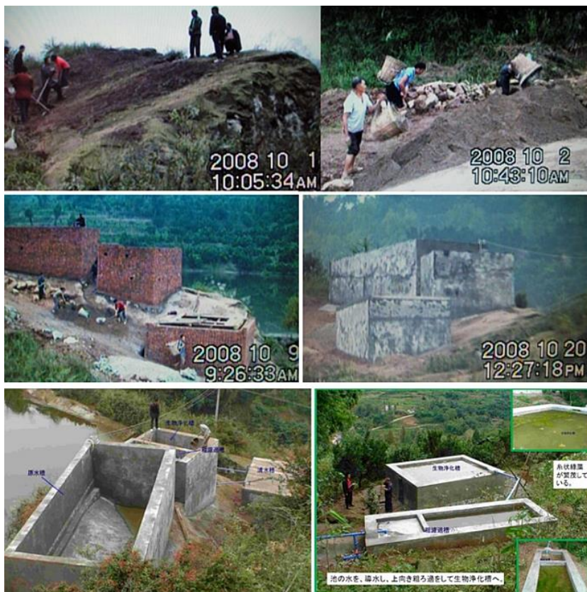
Fig. 18-2. EPS construction after the Great Sichuan earthquake
