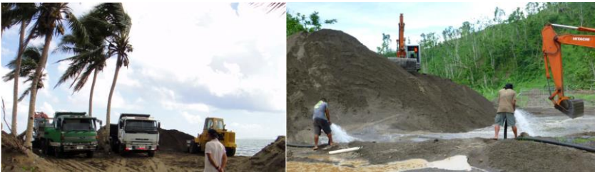
Fig. 16-4. Beach sand was taken and washed to put on the filter bed.
