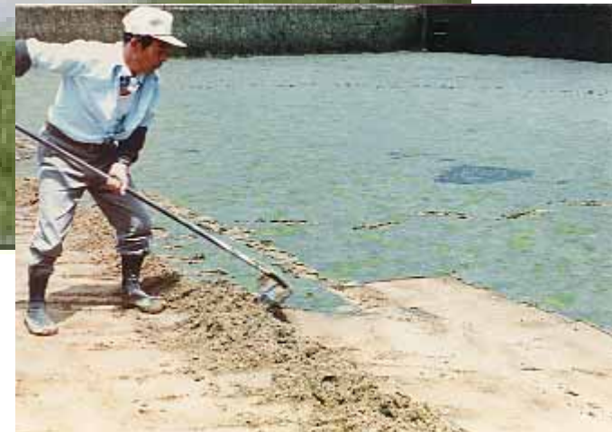
Scrapping of surface mud on the sand layer.
