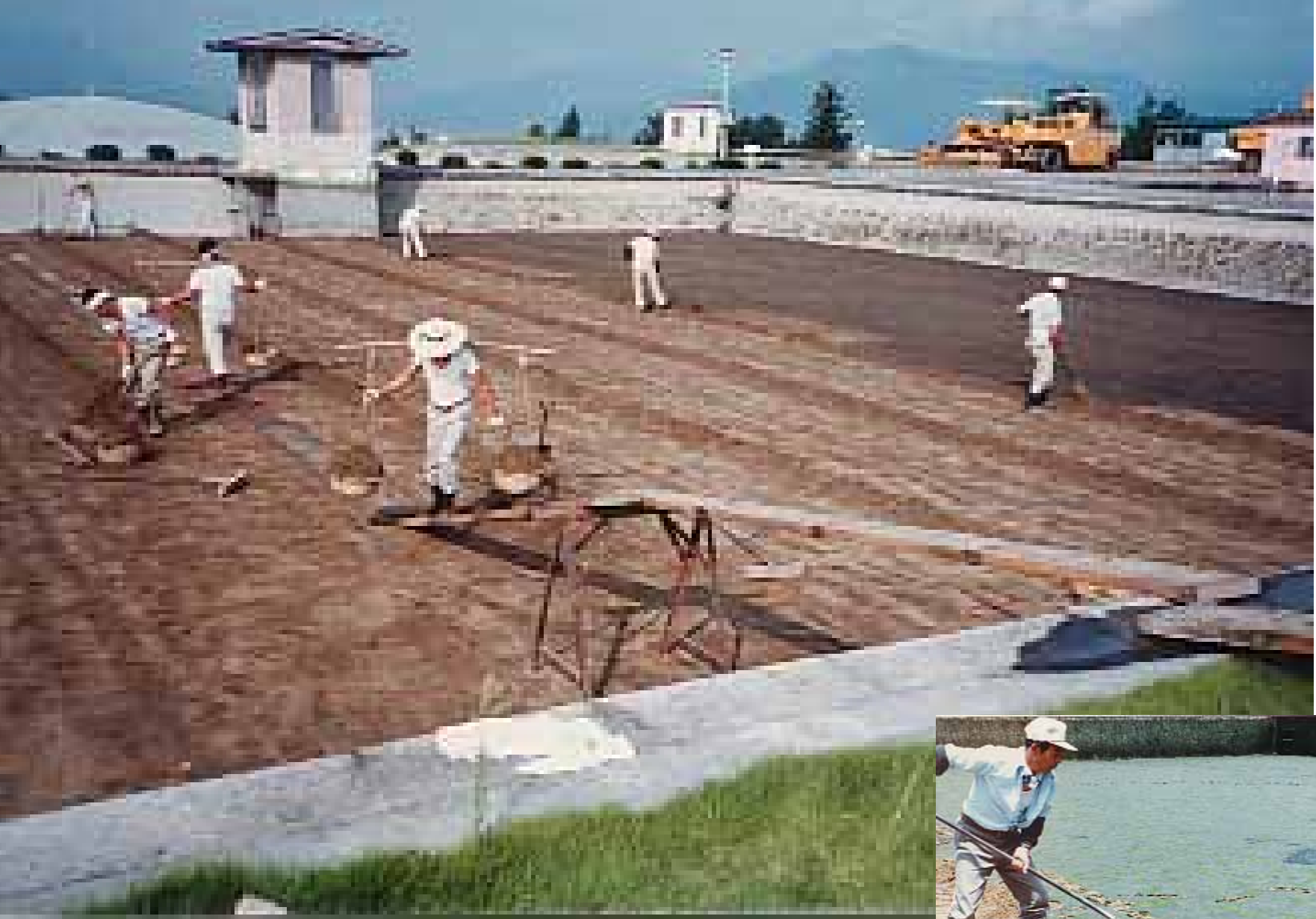
Scrapping of surface mud on the sand layer.
