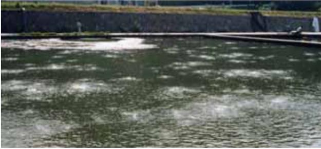
*There is super saturated condition of dissolved oxygen on the bottom by the activity of photosynthesis of the algal mat on the bottom. When the filter operation is suddenly stopped, so many bubbles are formed at the surface of the sand layer at that time. However, there is gentle water current during normal operation period. Small amount of oxygen bubbles are formed by the photosynthesis and these are trapped in the algal mat at the bottom.*
