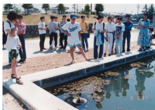
夏の上田市ではろ過開始後、糸状藻の連続培養系が約10日で成り立つ。 Continuous culture system of filamentous algae is observed in 10 days after a scraping.
